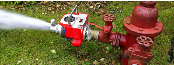
Fig. 1.3 Testing a pillar fire hydrant on a high pressure ring main
